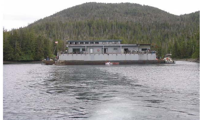
Crew barge 2007, south west shore of Kendrick Bay.
